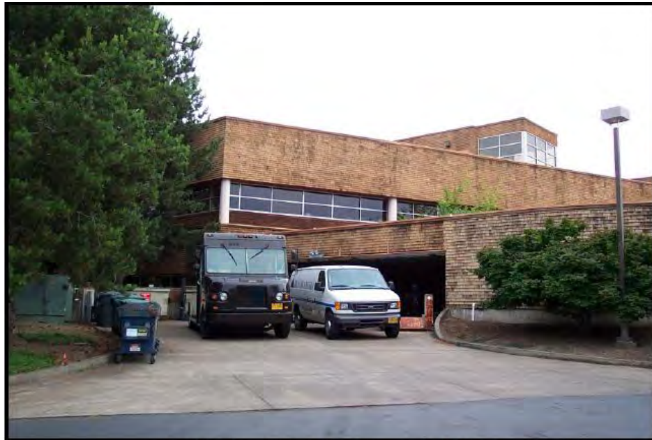
Loading Area at Southwest Corner of Building
