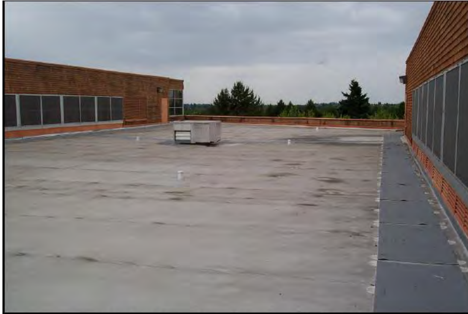
New Roof Cover (One of Four Sections of Building)
