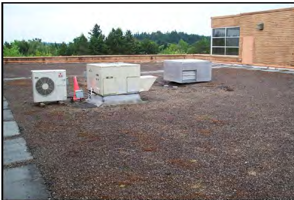
Original Roof Cover (Three of Four Sections of Building)
